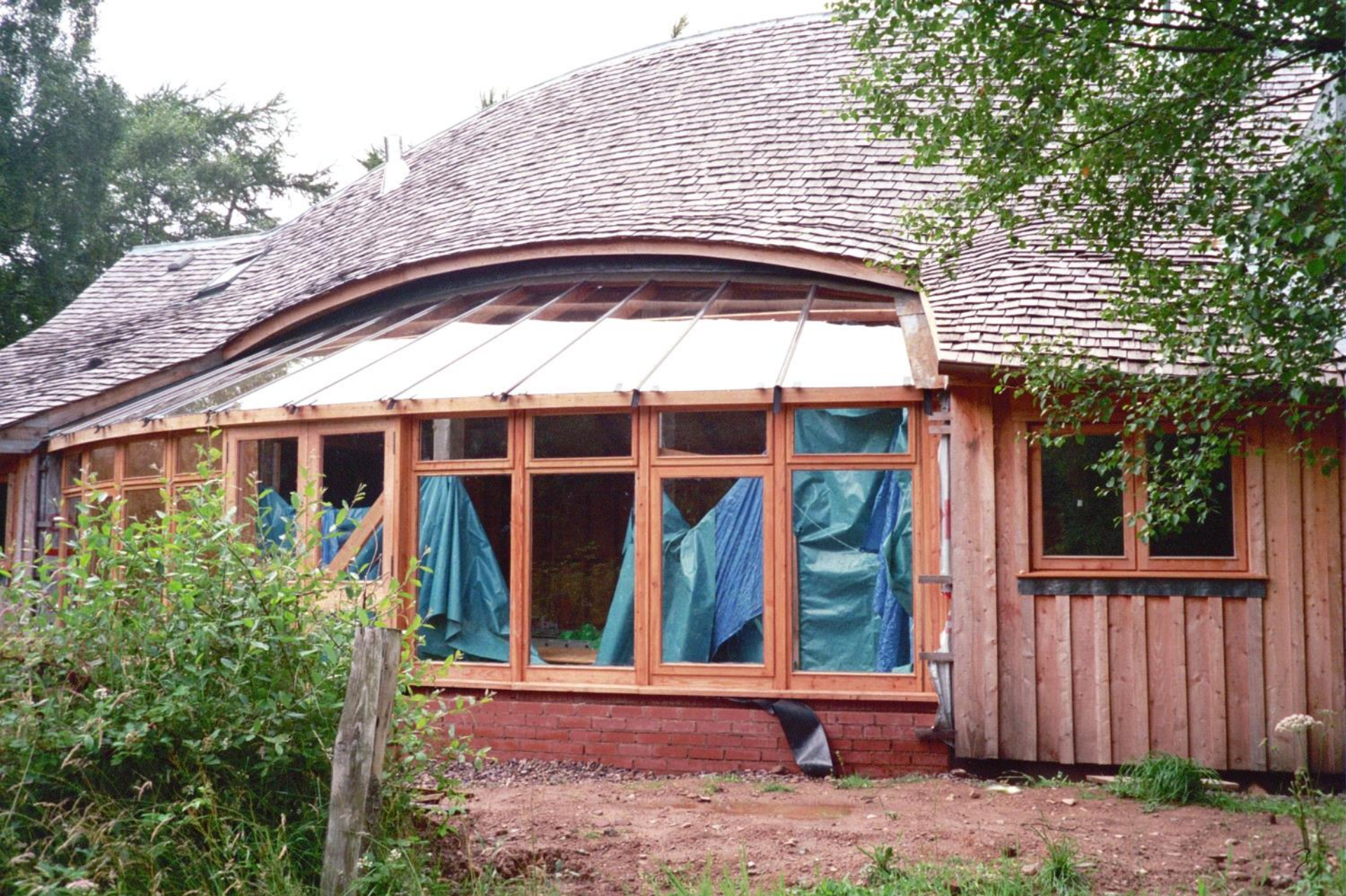
Solar heating by conservatory, 4 steps down
