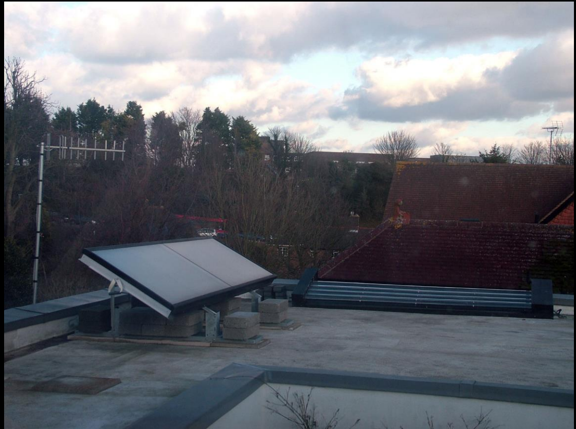
Atmos drain back solar thermal panel - N.B. spare one to rhs given away
