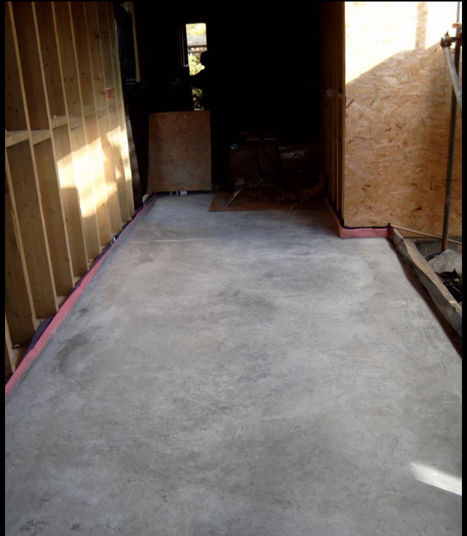
Power Floated 'heat sink' Screed finish with integral under floor heating
