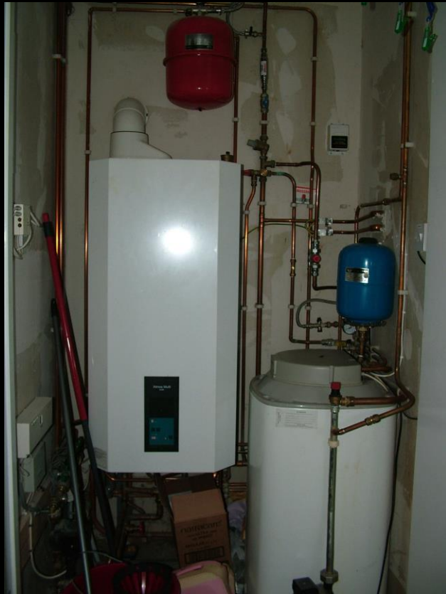
Atmos Condensing boiler with integral 80ltr tank & 110ltr solar store
