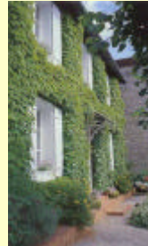
Fueullette House, Montargis, France 1921
