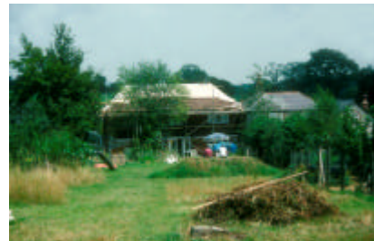
Repitching the roof. Note the Tyvek High Diffusive Roofing Felt.
