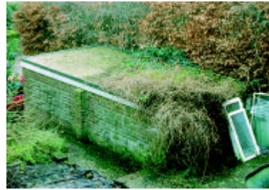
Eco-renovating a leaking tar and pitch roof.
