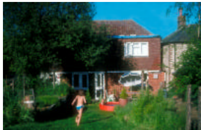
The old extension – drafty, subsiding and leaking water.
