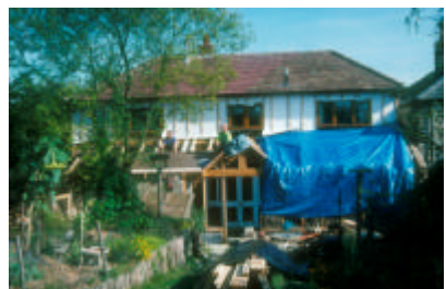
Passive solar conservatory and rear walls with 'breathing' membrane under construction.
