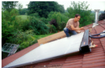
Installing the solar panel.
