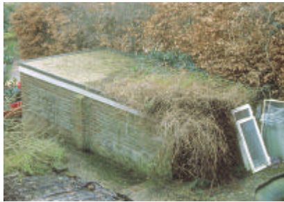
Eco-renovating a leaking tar and pitch roof.
