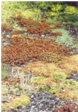
The sedum roof doesn't take long to establish and is popular with birds who forage for worms in the mulch material and collect nesting material in early spring.
