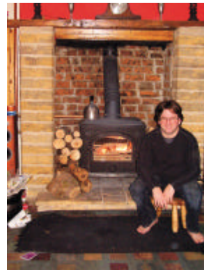
Andrew's Dunsleyheat Yorkshire stove is Clean Air Act exempt and heats both space (radiators) and water with its backboiler. It is backed up by the solar thermal panels.
