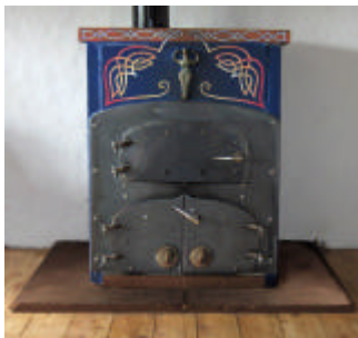
A masonry woodburning stove reduces gas and oil bills. This example is home made out of paving slabs.
