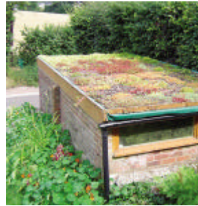
After stripping the roof, we laid a membrane over the existing chipboard, added sifted top soil & planted drought resistant sedum.
