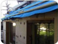
External Insulation - Eaves and window reveals: The external insulation is fixed back to the structure by way of plastic headed ficings.
