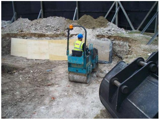
With the help of Apprentices The Mears Group compacted existing ground to act as ground slab to reduce concrete and avoid spoil leaving site
