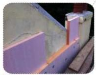
Section Detail - Basement window head: The external insolution is fixed in panels and may be made up of several layers depending on the u-value required and the associated thickness.
